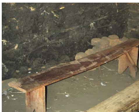
Mud and stick walls, dirt floor and a bench for little backsides 2009. This resembles the old classrooms in the first building, but is where the children study in what was the store room.
